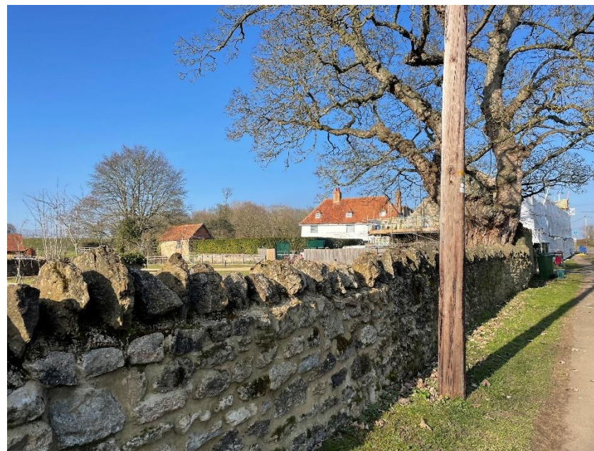
Plate 30 View of Park End looking north along Kennington Road – listed barn is visible but was covered in scaffolding at time of site visit
