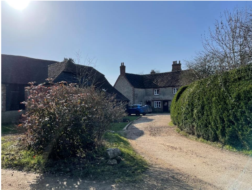
Plate 23 Lower Farmhouse, looking southwest
