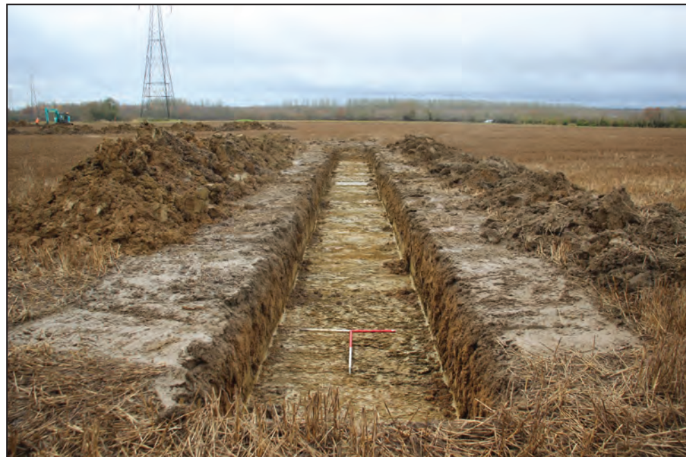
Trench 25, looking west (1m scales)
